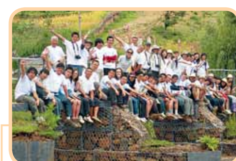
Wu Zhi Qiao (Bridge in China) Bridge building project of the Paomapi village in Yunnan
